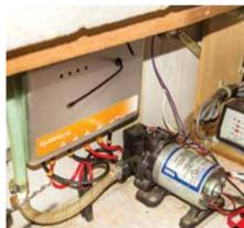
**10.** An isolator switch needs to be mounted in-line with the battery and the ECU, so the unit can be manually switched off. Find a suitable location near the battery, and run the power from the battery, to the isolator, and then to the ECU ensuring all cabling has been insulated in flexible conduit for additional protection.
